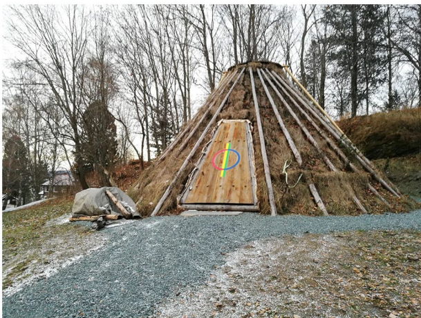
Figure 2. The door in place and the roof hatch (Photograph: Asbjørn Kolberg).
